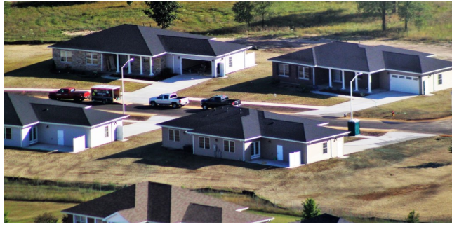
Construction of new military family housing at Fort McCoy
