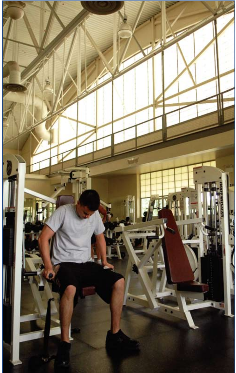
High-efficiency windows in the gym at Barksdale AFB provide natural light while preventing heat transfer, helping to save electricity on both lighting and air conditioning.
