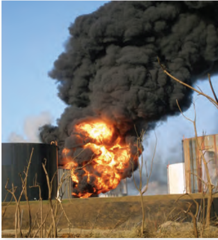
When this fire and ensuing explosion near an Army installation damaged Army facilities last year, the Region Director convened a crisis action team, dispatched an assistance team to the garrison and re-directed assets for recovery operations.
