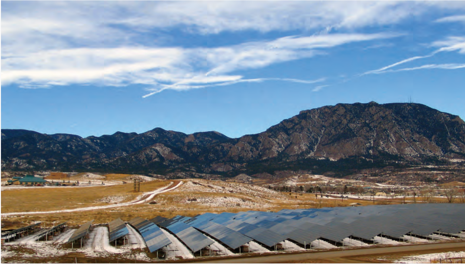
The Fort Carson, Colo., Solar I, a 2-megawatt photovoltaic array, was completed in December 2007. The 15-acre array, located on a former construction debris landfill site, generates approximately 3,200 megawatt-hours of power annually.
