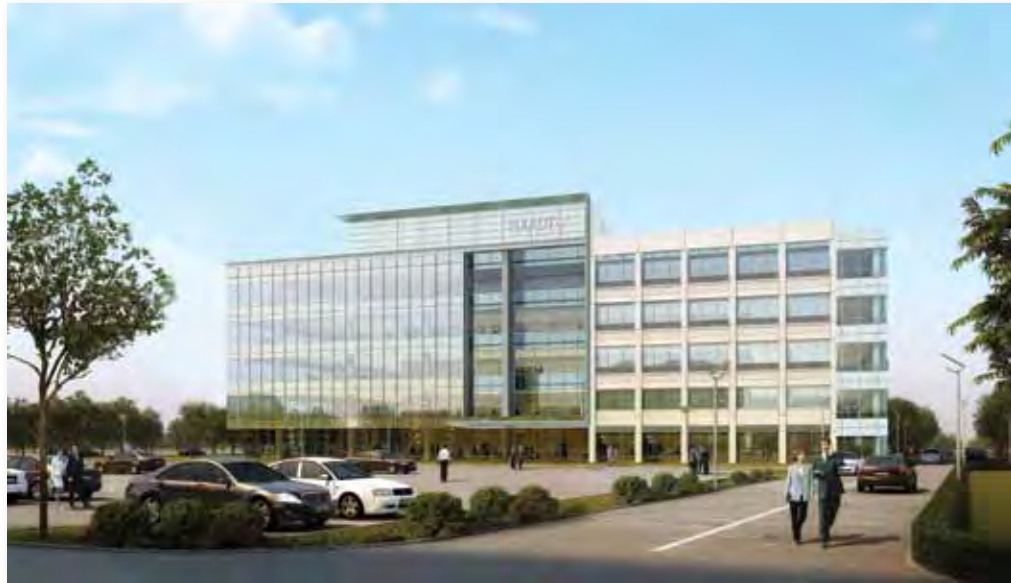
An artist rendering of the first building under construction at Redstone Gateway with construction of this building expected to be complete by November 2011. At full build-out, Redstone Gateway will have over 4.6 million square feet and will house a combination of administrative, research and development, academic and retail space.
