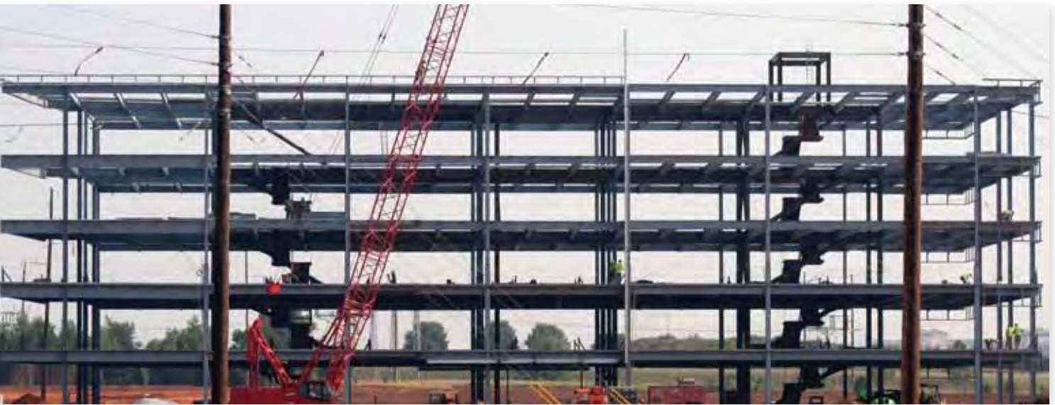
Ongoing construction for the initial building in the Redstone Gateway office park. This Enhanced Use Lease project is the result of the partnerships between Redstone Arsenal, the city of Huntsville, Madison County and state officials as well as the development team of COPT and Jim Wilson & Associates.
