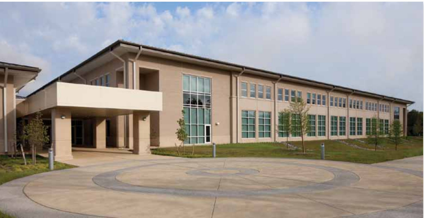
Joint Strike Fighter (JSF) Academic Center at Eglin Air Force Base, Florida. The JSF initial joint training site will support 1,900 military personnel and over 400 contractors.
