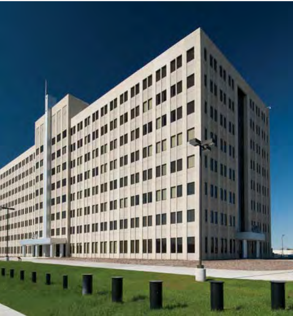
The LEED Silver BRAC administrative building at the U.S. Army Garrison - Detroit Arsenal was completed nearly $30 million under budget, cost overruns were kept to less than two percent and the building was completed three months ahead of schedule.
