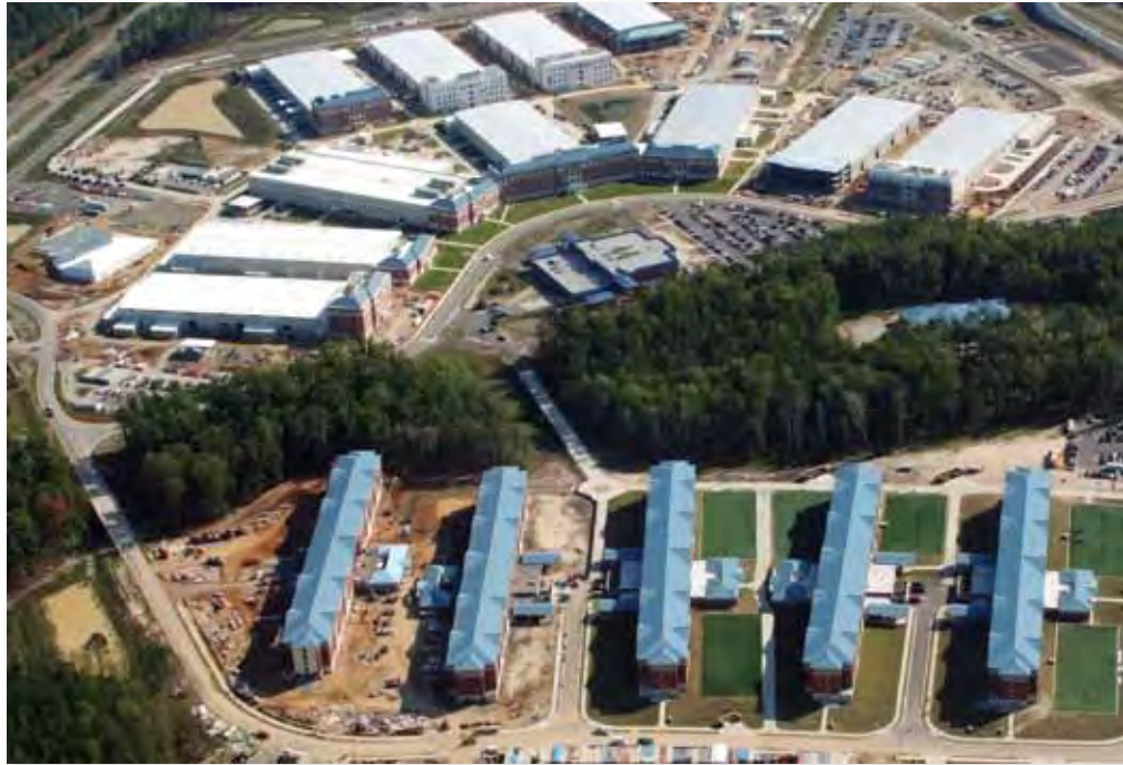
The Army's new Ordnance School campus is located north across Route 36 from the main portion of the Fort Lee installation, significantly increasing the footprint of the post's training facilities. (U.S. Army photo by Albert Cruz)
