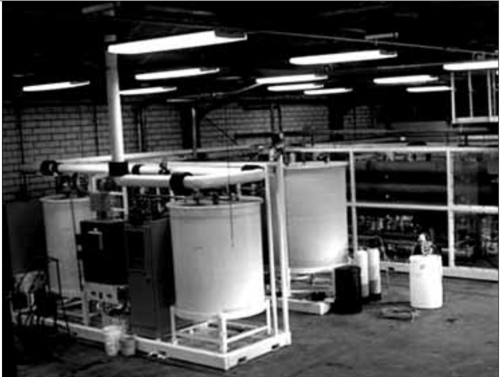
Supercritical Water Oxidation System (SCWO): In FY06, the SCWO at McAlester Army Ammunition Plant, OK, will support demil by converting hazardous chemicals and materials into benign compounds using water at high temperatures and pressures.
