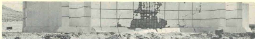
MODEL STRUCTURE, designed to resist effects of accidental explosion, is shown after tests with 2,000 and 3,500 pounds of high explosives by Picatinny Arsenal.
