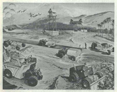
FAMECE, denoting Family of Military Engineer Construction Equipment, is being developed by the Mobility Equipment R&D Center to increase mobility of earthmovers and decrease the logistical burden caused by multiplicity of makes and models in the field. FAMECE features a common mobile power module that will accommodate as many as 13 different pieces of construction equipment.
