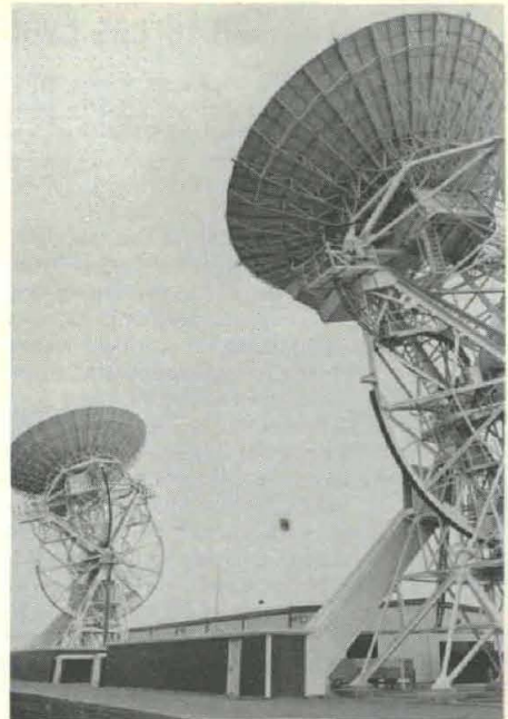
TWIN 60-foot satellite antennas track orbiting Soviet MOLNIYA communications satellites and provide a U.S. terminus for the Direct Communications Link.
