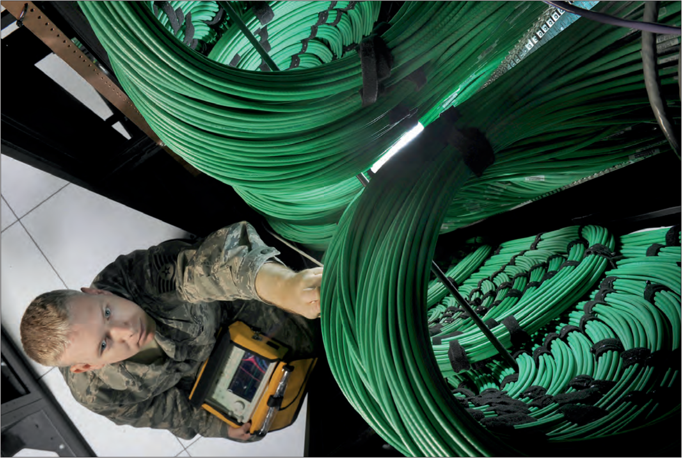
Airman uses spectrum analyzer to check television broadcast network routers (U.S. Air Force/Val Gempis)
