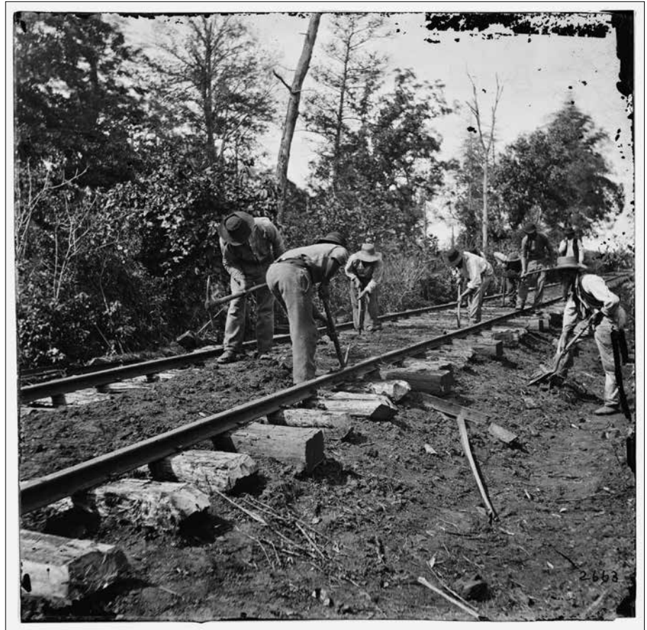
Men repairing single-track railroad near Murfreesboro, Tennessee, after Battle of Stone’s River (LOC)
