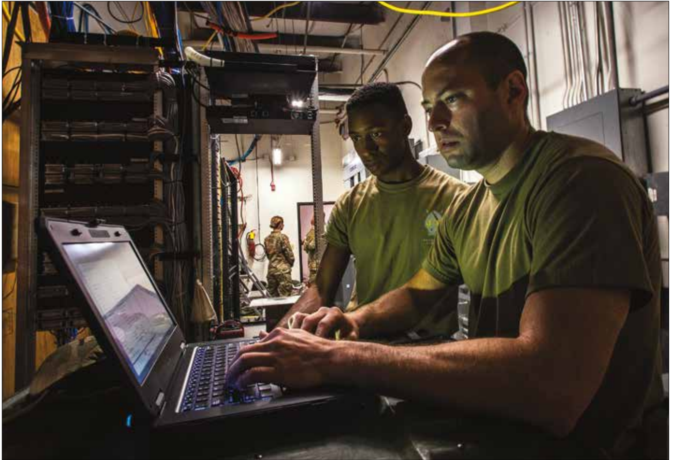
South Carolina Army National Guardsmen from 228 th Signal Brigade out of Spartanburg, South Carolina, set up Joint Incident Site Command Center package to support Horry County Emergency Operations Center with back-up communications system, September 15, 2018 (U.S. Army National Guard/ Brian Calhoun)
