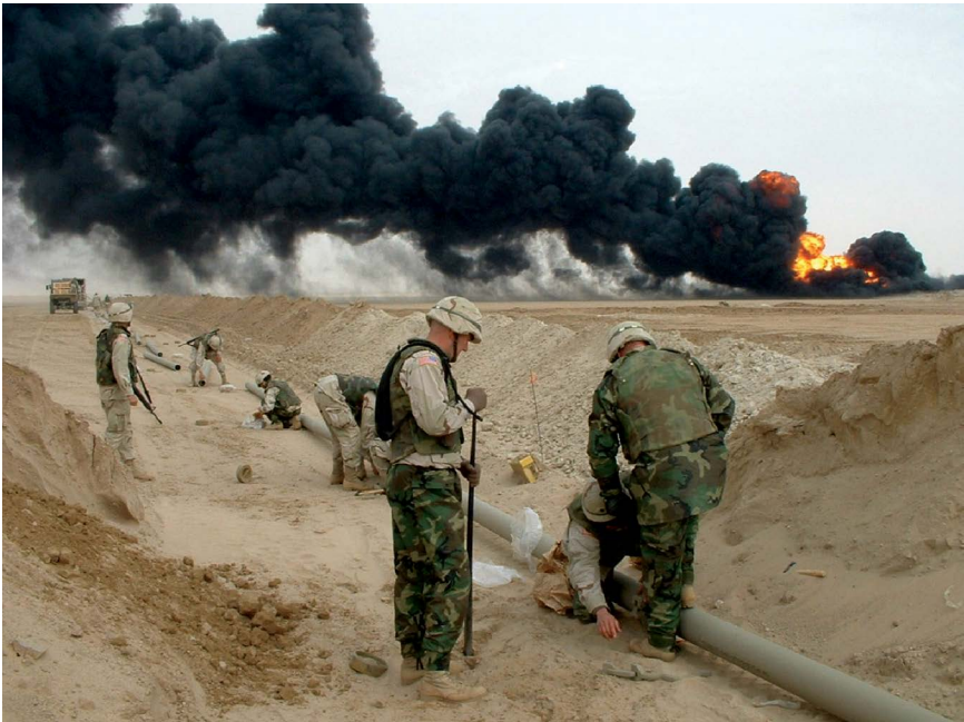
Figure 11.4. The installation of the IPDS into Iraq slowed the rate of construction as the troops worked in the debilitating heat wearing full combat equipment. Despite this, throughout OIF I, the rate of construction exceeded the doctrinal standard. Photo courtesy of 416th Engineer Command.
